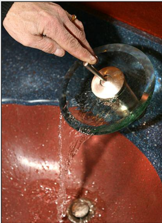
New faucets were installed in the ladies' room.
