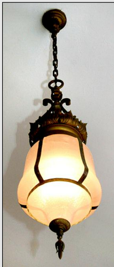
One of the new lights in Lodge Room No. 1.
