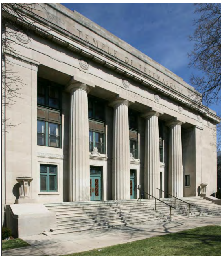
Madison Masonic Center, 301 Wisconsin Ave., Madison. Photo by Rich Rygh
