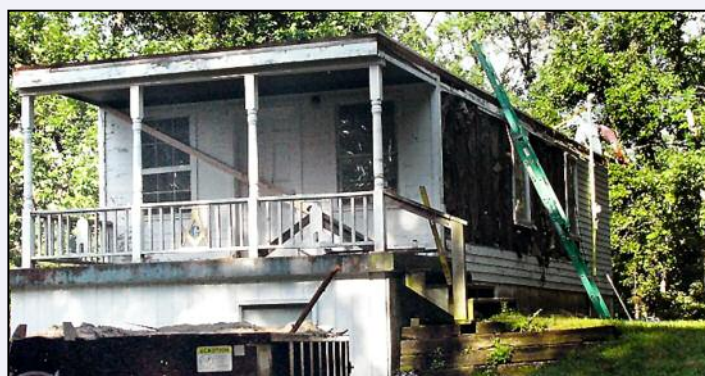
Lodge building during the remodeling.
