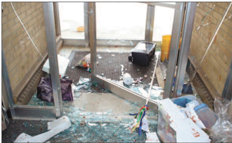
North entrance to the building.
