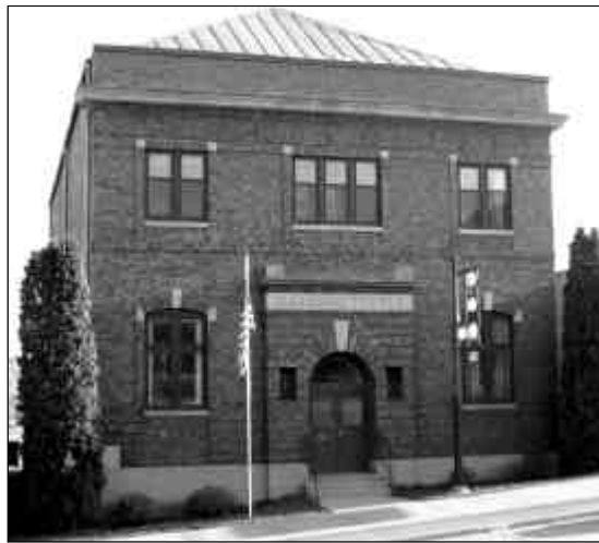
Black River Lodge Features a new metal roof and refurbished lodge room. The lodge will be rededicated in a program June 24.
